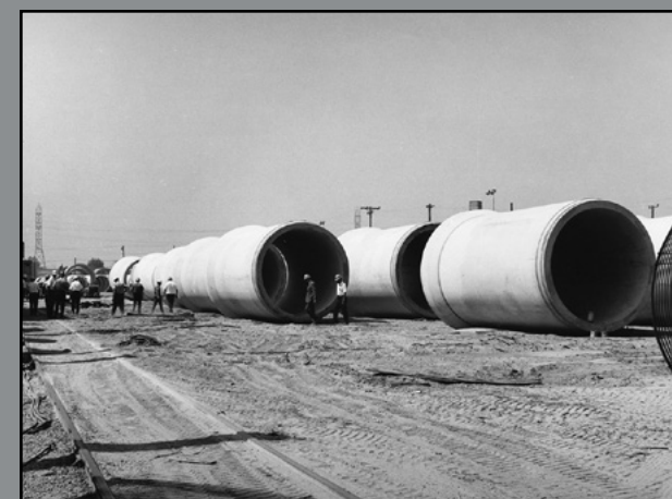
Ocean outfall pipes, circa 1970s
