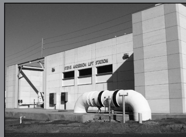
Steve Anderson Lift Station, circa 2009
