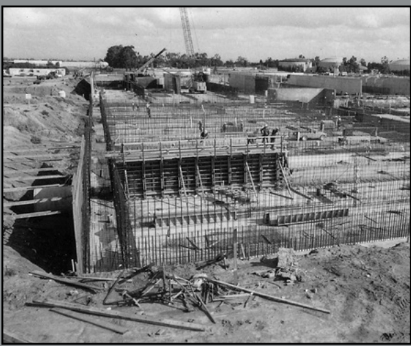
Construction of Activated Sludge Facility at Plant No. 1, circa 1978
