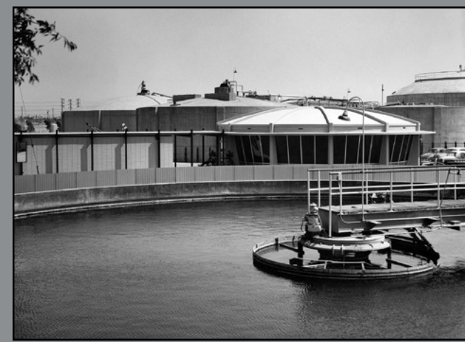
Original Control Center and clarifier at Plant No. 1, circa 1957
