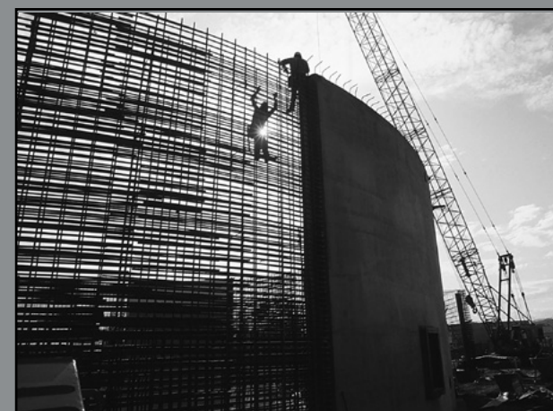
Construction of trickling filter at Plant No. 1, circa 1991
