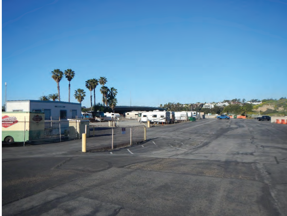
Photograph 3 – View of the project site, an parking lot and storage facility at the site of the existing and proposed pump stations, facing west.
