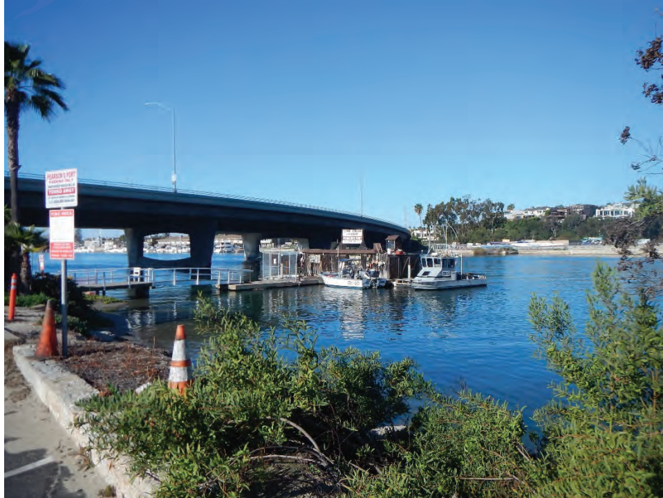
Photograph 4 – View of the Bay Bridge (PCH) and Newport Bay north of the PCH, facing southwest.
