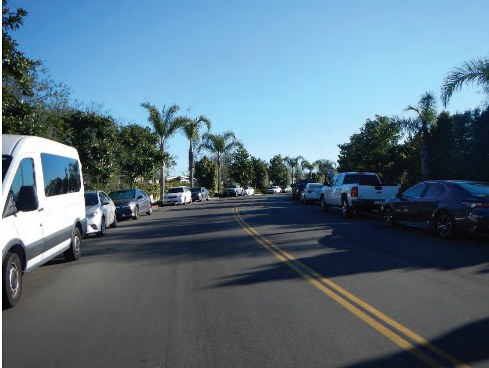
Photograph 2 – View of Bayside Drive north of the PCH within the project site, facing north.
