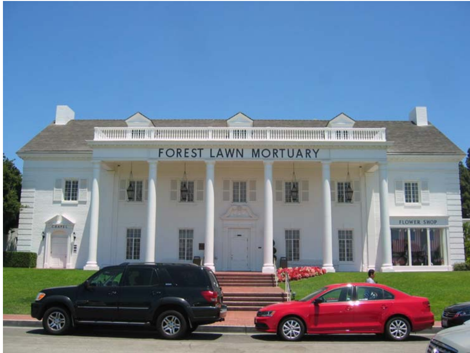
Figure 12. Main mortuary building, view to north. June 25, 2015.
