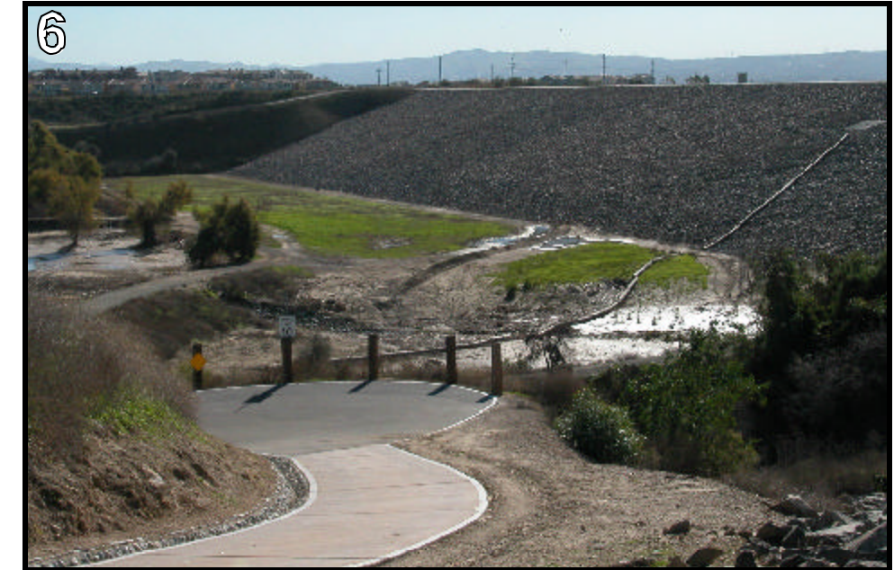
View from the west of the Carbon Canyon Dam basin.
