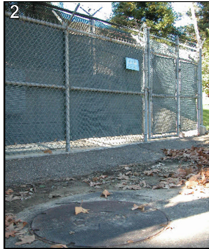
The existing Carbon Canyon Pump Station. The proposed pipeline begins at the manhole visible in the foreground.
