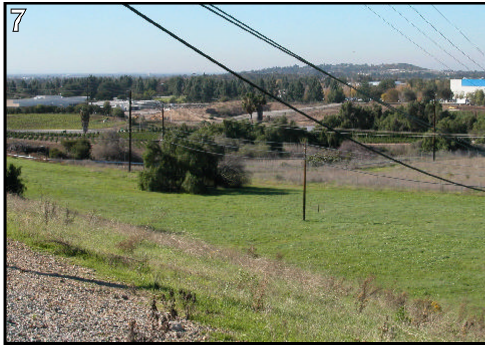
View from the northeast of the intermediate jacking pit area as shown in Exhibit 3.0-3.
