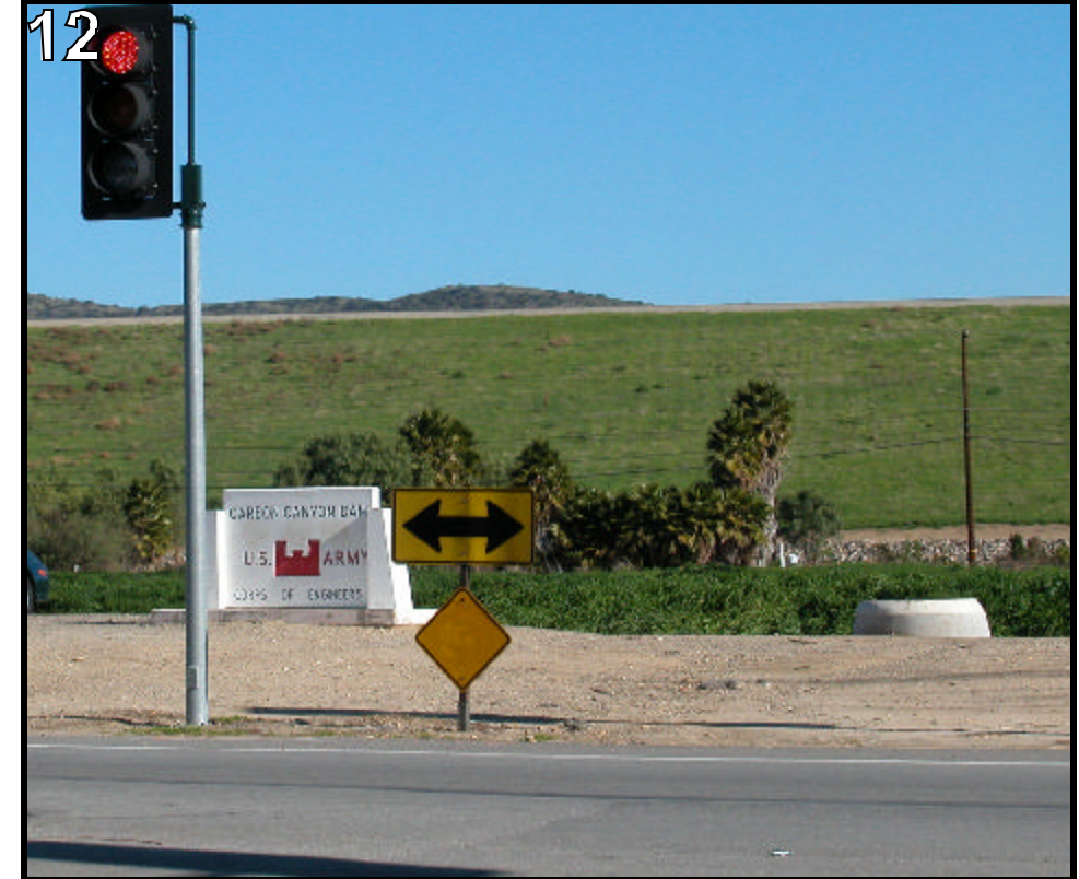
View from the southwest of the intersection of Rose Drive and Vesuvius Drive, where the proposed pipeline would connect with the Carbon Canyon Interceptor. Carbon Canyon Dam is in the background.
