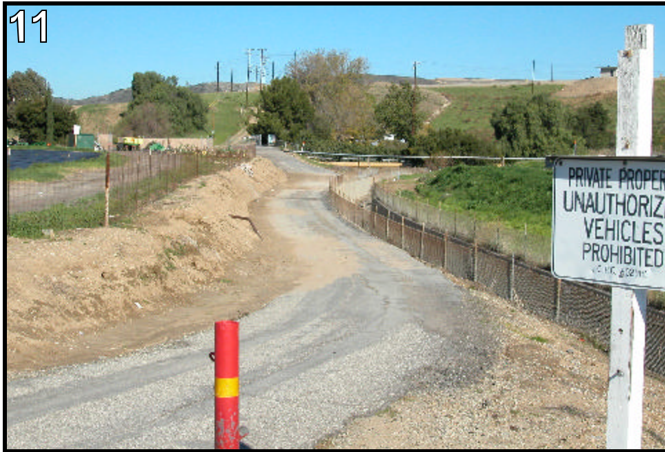
View from the southeast of the existing U.S. Army Corps of Engineers access road the proposed pipeline alignment would follow prior to connecting with the Carbon Canyon Interceptor.
